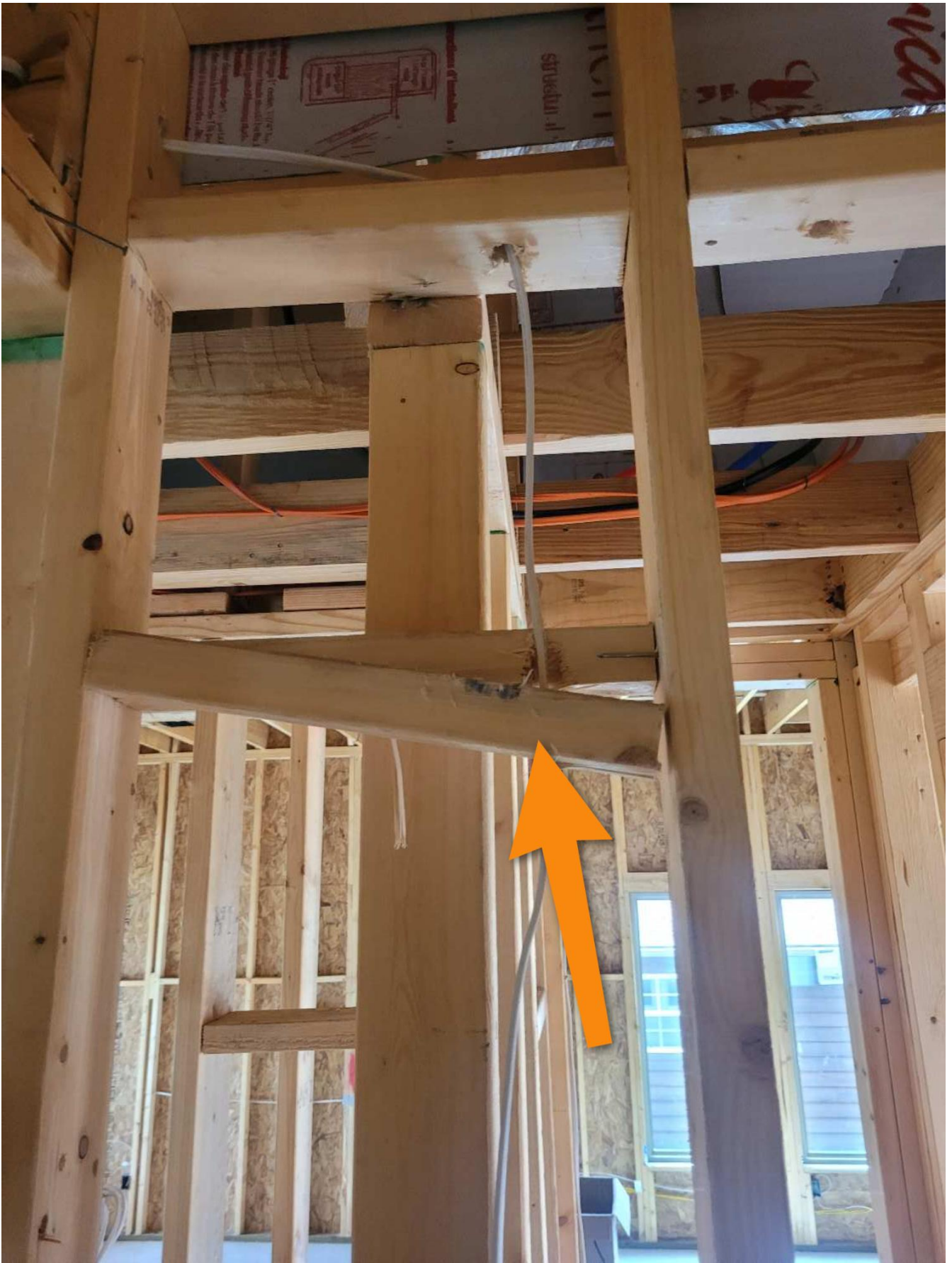
Damaged Blocking
